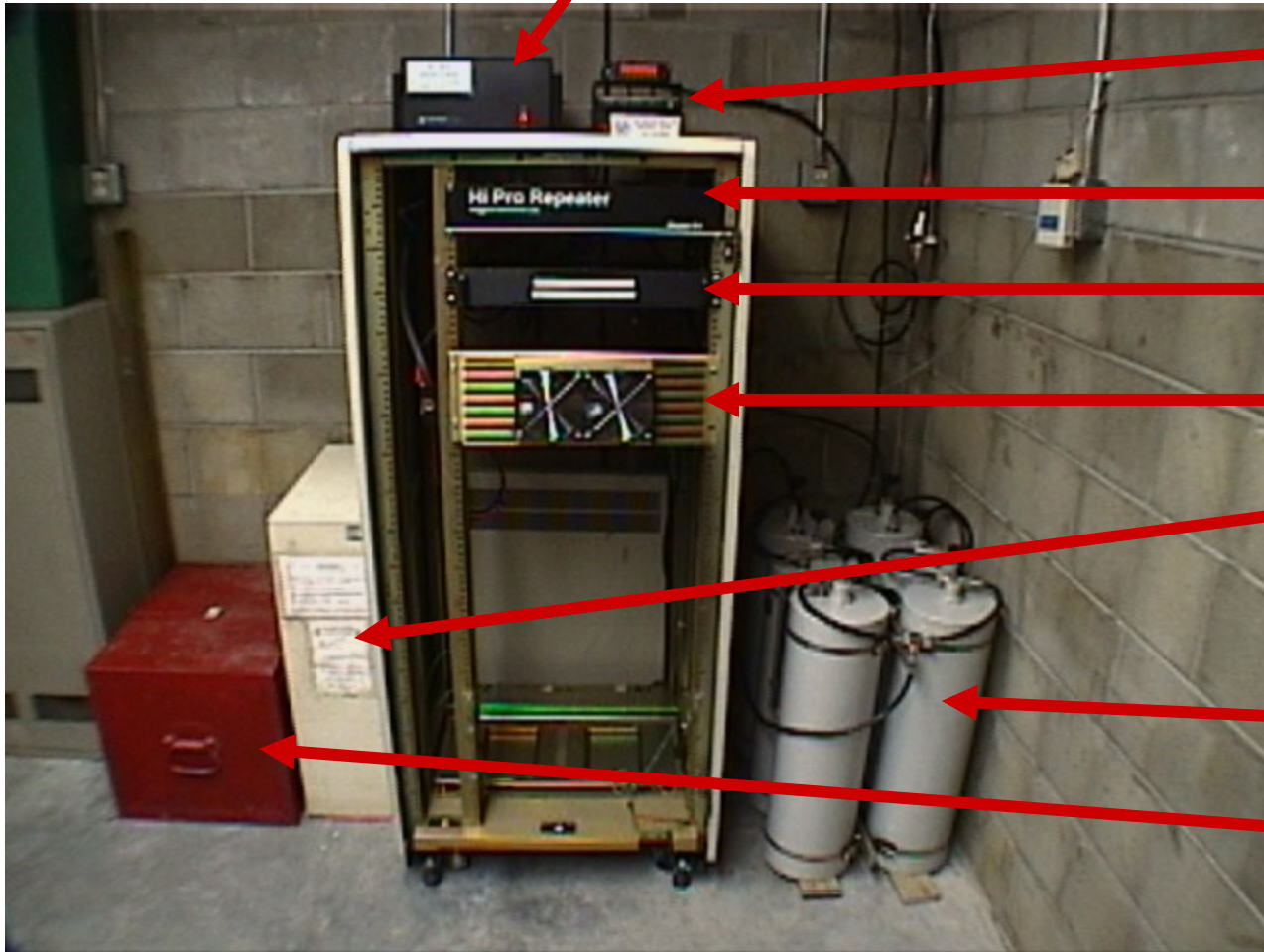
WTRA RACES District 10 Repeater, Duplexer, Packet Node, and Remote Base - Equipment Installation
